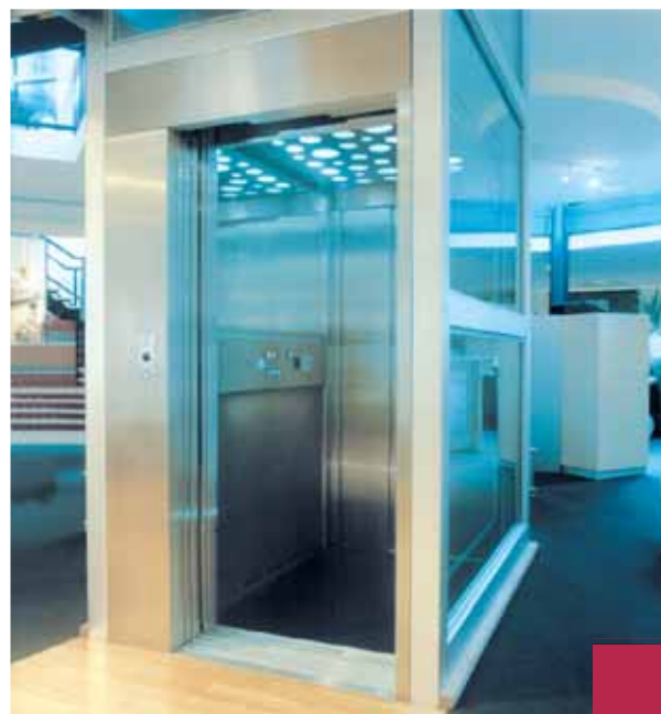
Installation in a furniture shop (The Netherlands), white painted structure supported frame, glass cladding and car with stainless steel finishes.
