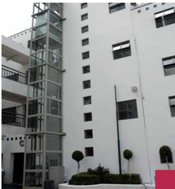
Outdoor installation in a condominium (Mexico), structure cladding in glass. Thanks to the structure supported frame, the lift can be installed also without a dedicated shaft.
