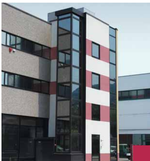
Installation in a company (Italy), black painted structure supported frame with mirror glass cladding.
