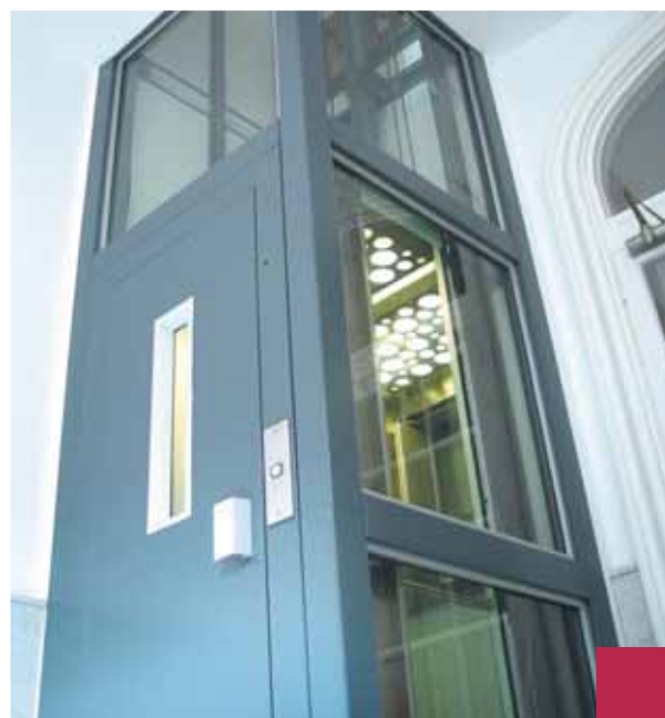
Installation in a private house (The Netherlands), indoor structure supported frame, glass cladding, car with panoramic wall and hinged door with window.
